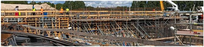
Concreting of the foundation slab of one of the two newly-built CCGT units in the Dolna Odra Power Plant, a company branch of PGE Górnictwo i Konwencjonalna which belongs to PGE Group, has been completed. The construction of low-emission units with a total capacity of 1340 MW is a strategic project for the Polish economy.
