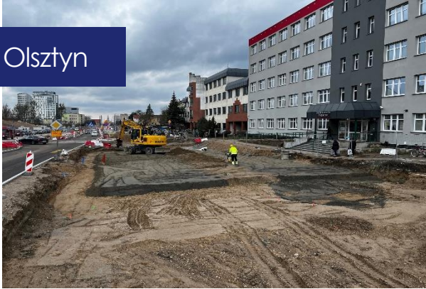
Extension of tram network in Olsztyn
