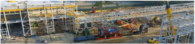
The foundation of the steam turbine at the construction site of the New Czechnica Combined Heat and Power Plant is ready. Installation of the first pieces of process equipment including the four peaking and reserve boilers begins. The construction of a gas-fired combined heat and power plant in Siechnice near Wrocław is a priority investment by Zespół Elektrociepłowni Wrocławskich KOGENERACJA S.A., part of the PGE Energia Ciepła Group.
